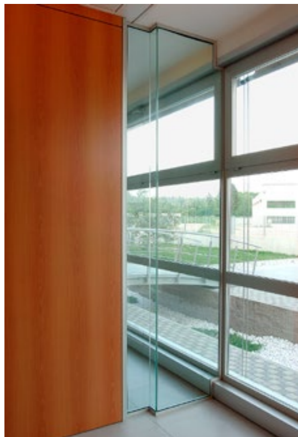
Fissaggio a parete e serramento Fixing to wall and building frame
