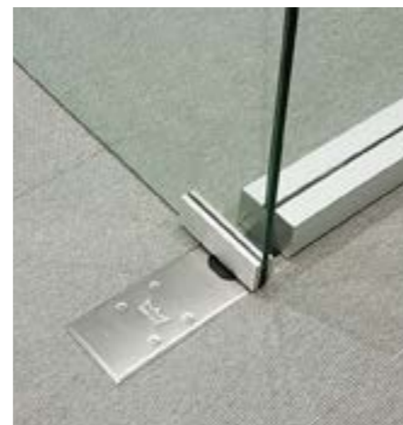
Cerniera a pavimento Hinge at floor level
